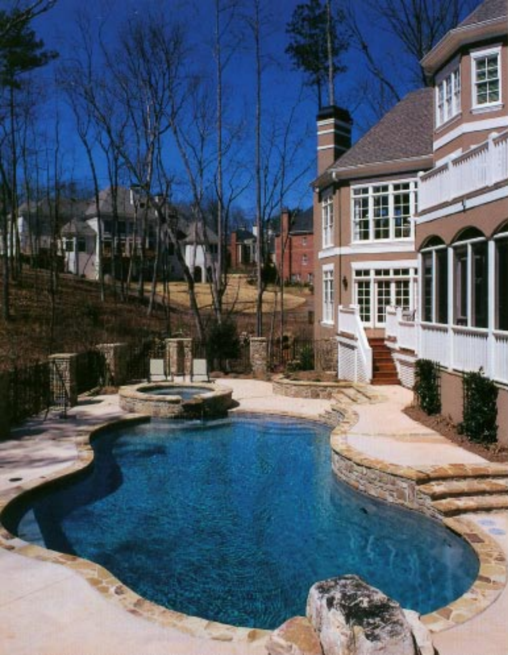
Tom Eldridge's attention to fine detailing is evidenced not only in the front of the home, but in the back elevation as well. Here, a screened-in porch and second floor balcony overlook an inviting free-form pool and hot tub. Photography by Bryan L. Willy, Willy Photography.
